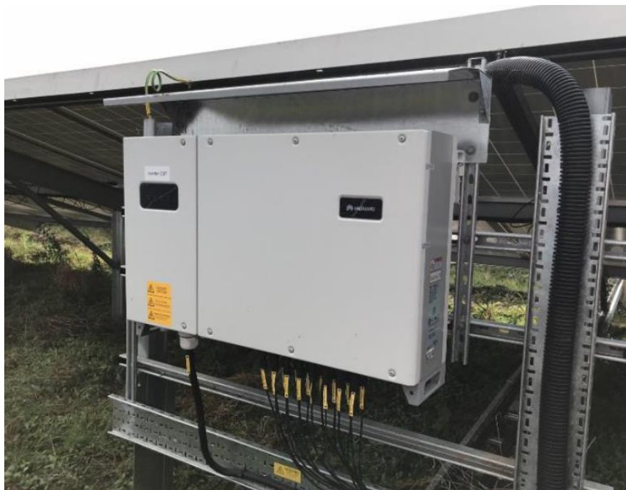
Figure 2.2 Typical String Inverter (image reproduced courtesy of Huawei)
